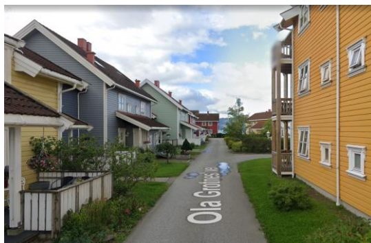
Figur 4-10: Rekkehus (Google Maps)
